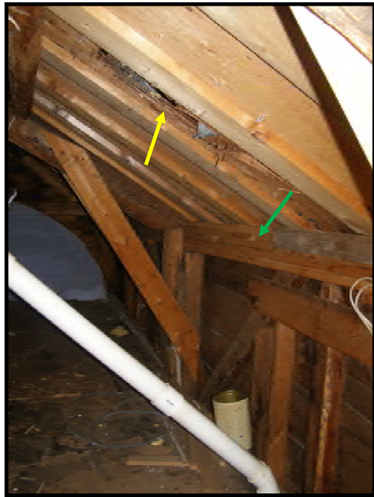
Easterly eave space at second story of Masonic Temple. The yellow arrow is indicating a hole in the OSB roof sheathing. Additional diagonal bracing has been added to the bent framing between the post and rafter. A section of the top plate has been replaced with dimensional lumber (green arrow).
