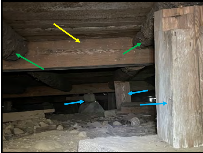
Masonic Temple crawl space/floor system. Yellow arrow indicates main carrying beam (with powder post beetle frass). Green arrow indicates 3/4 timber joists. Wood post and stone piers can be seen in this photo, supporting both beams and bolstering joists, (blue arrows).
