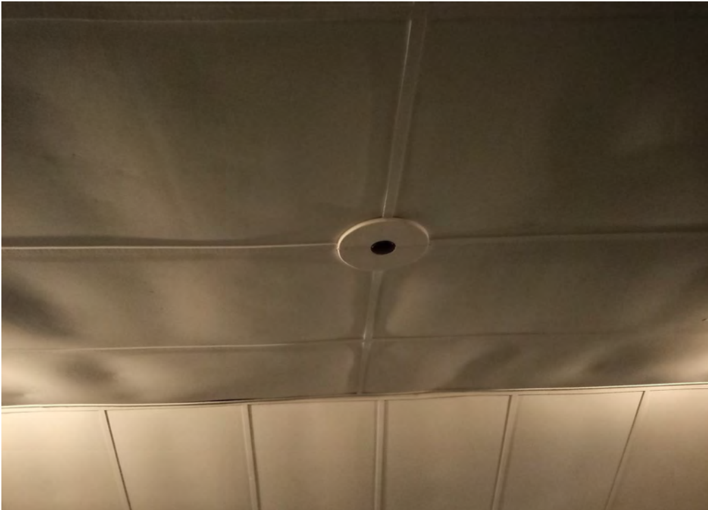
Figure 120: Cupping and bubbling at second floor ceiling, possibly due to moisture or water infiltration
