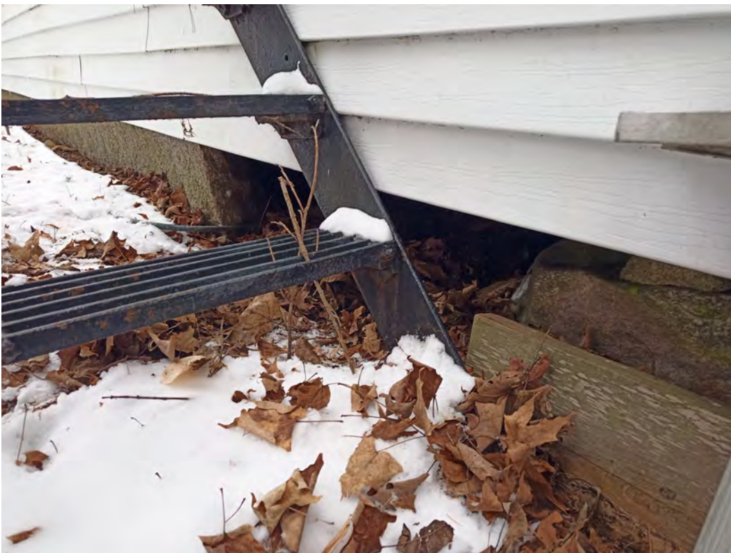
Figure 84: Displacement and cracking at split-granite stones, typical
