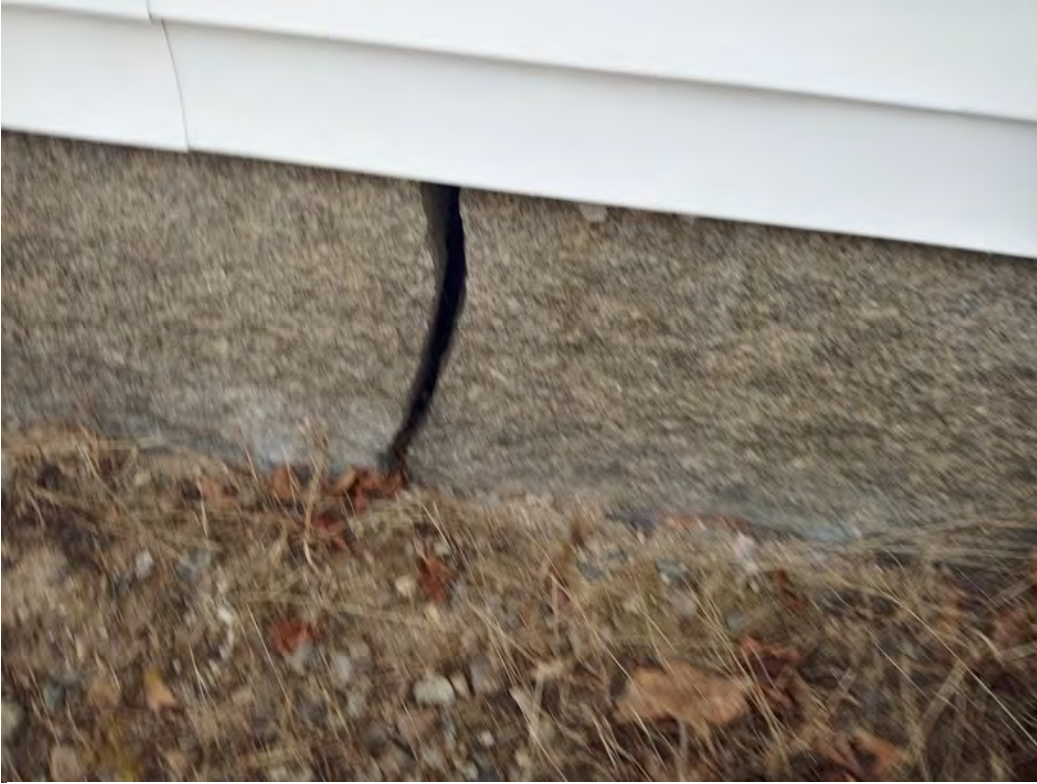
Figure 87: Cracking through split-granite foundation stone
