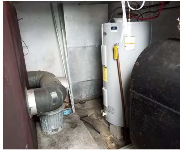
Figures 136-141: From top left to bottom right: Thatcher furnace, oil tank, hot water heater, large rigid metal ductwork, sole main hall heat supply register
