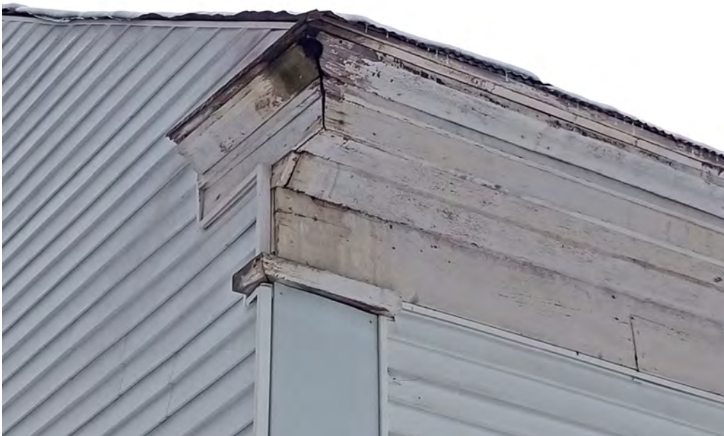
Figure 103: Intact wood cornice / eave trim; Cracking, material loss (hole likely due to squirrel entry), and worn paint observed, typical.
