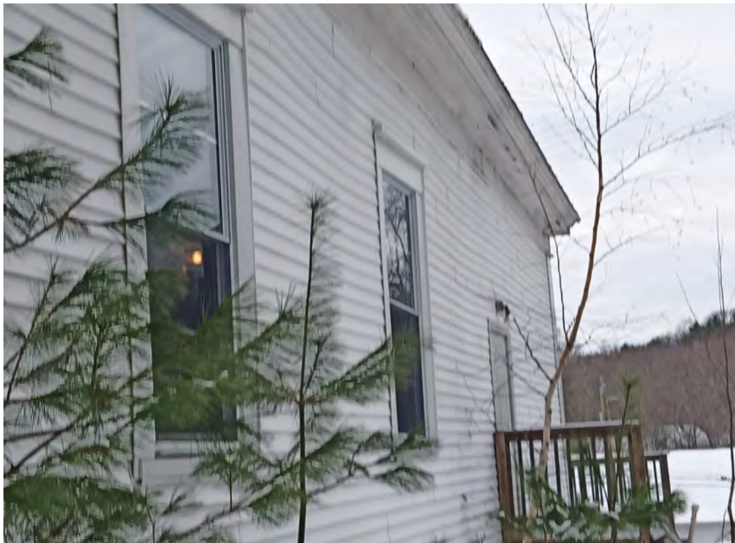
Figure 105: West façade vinyl-covered clapboards exhibit waving. Upon removal of vinyl, portions of clapboards may need to be resecured to framing. Remove tree growth at building perimeter.
