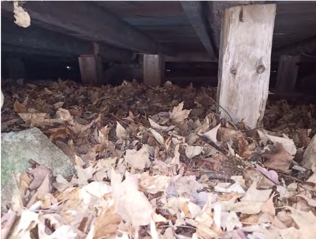
Figure 85: Debris accumulation in crawlspace. First-floor beams supported on dry-laid stone, joists reinforced with wood posts throughout. Check and supplement posts regularly, and as needed.
