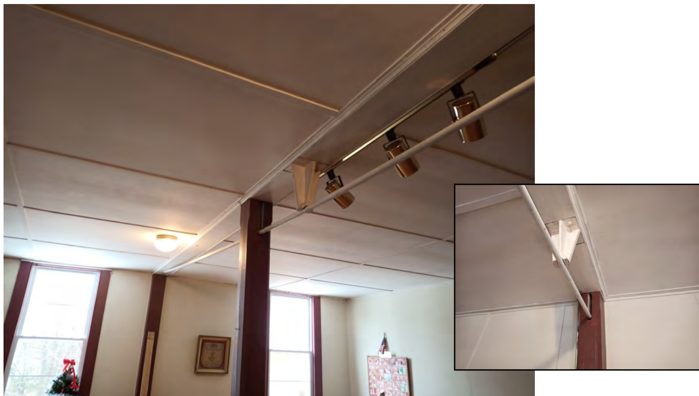
Figure 57: Main Hall ceiling; Inset: Tension rods
