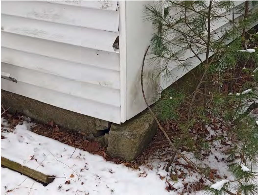
Figure 80: Displacement and cracking at split-granite stones, typical
