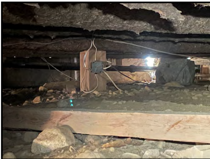
Masonic Temple crawl space/floor system. The condition of the crawl space is quite good, dry with sufficient space between the dirt floor and undersides of the wood floor members. This photo also shows an electrical junction box with exposed and unsupported non-metallic wiring.
