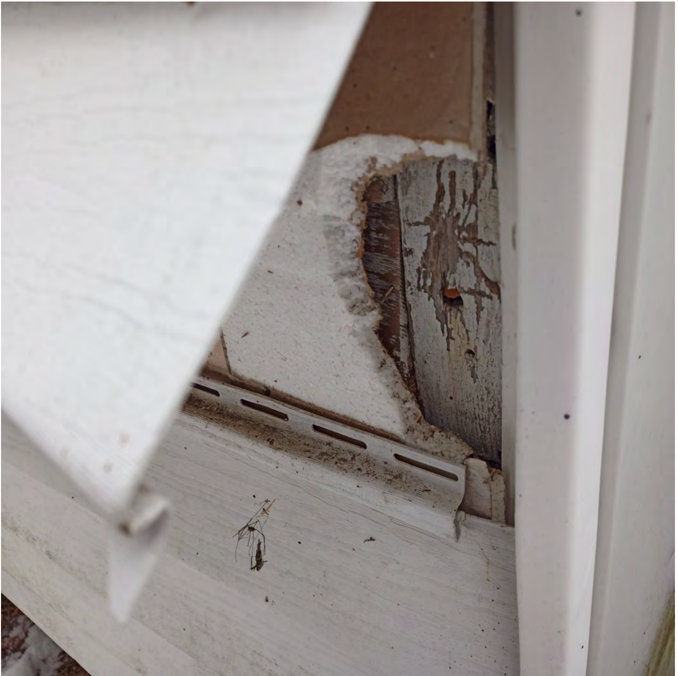
Figure 100: Vinyl siding lifted to reveal intact wood corner board and clapboards
