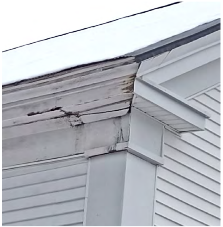
Figure 102: Intact wood cornice / eave trim; Cracking and worn paint observed, typical.
