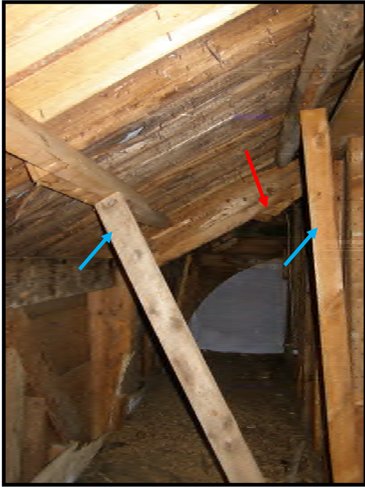
Westerly eave space at second story of Masonic Temple. Evidence of the original arched ceiling can be seen at the end (gable) wall. The original collar tie joint at a bent can also be observed (red arrow). This side of the roof remains sheathed in 1x boards. Additional dimensional lumber bracing has been added to support the roof purlins (blue arrow)
