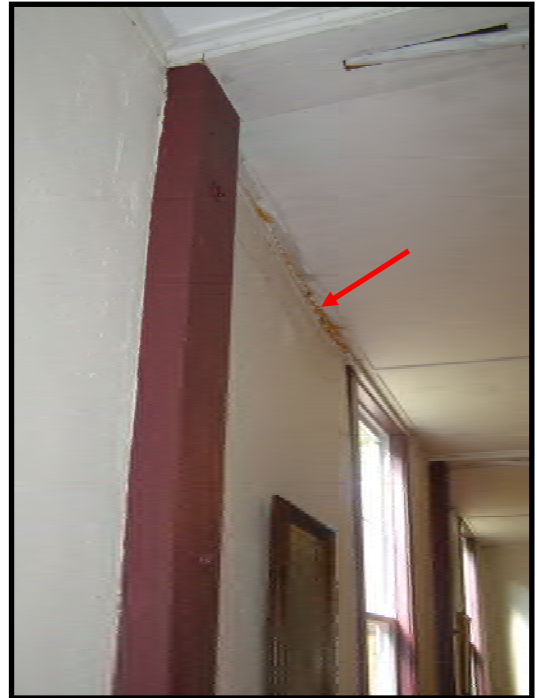
Westerly exterior wall of the Masonic Temple, viewed from inside the banquet hall. Signs of wall splaying can be observed at the wall-ceiling intersection.
