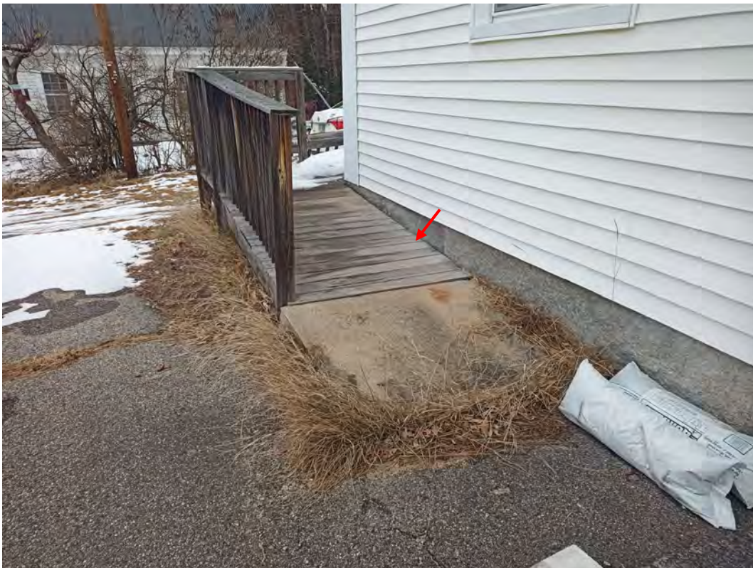
Figure 77: Accessible ramp butts up against building wall resulting in moisture accumulation along joint
