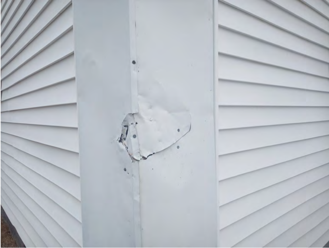
Figure 106: Damage at southeast vinyl corner trim
