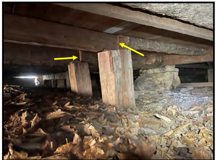
Masonic Temple crawl space/floor system. Yellow arrow indicates where timber joists have been cut/removed and replaced, with new wood posts installed at the joint. Wood posts have moved out of plumb, likely a result of seasonal movement over time.
