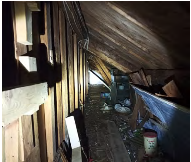
Figures 126-130: First floor tension rods, attic roof timbers, cut collar ties.
