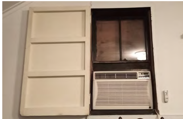
Figure 112: Sheathed over rear window with 1926-era 2/2 sash intact
