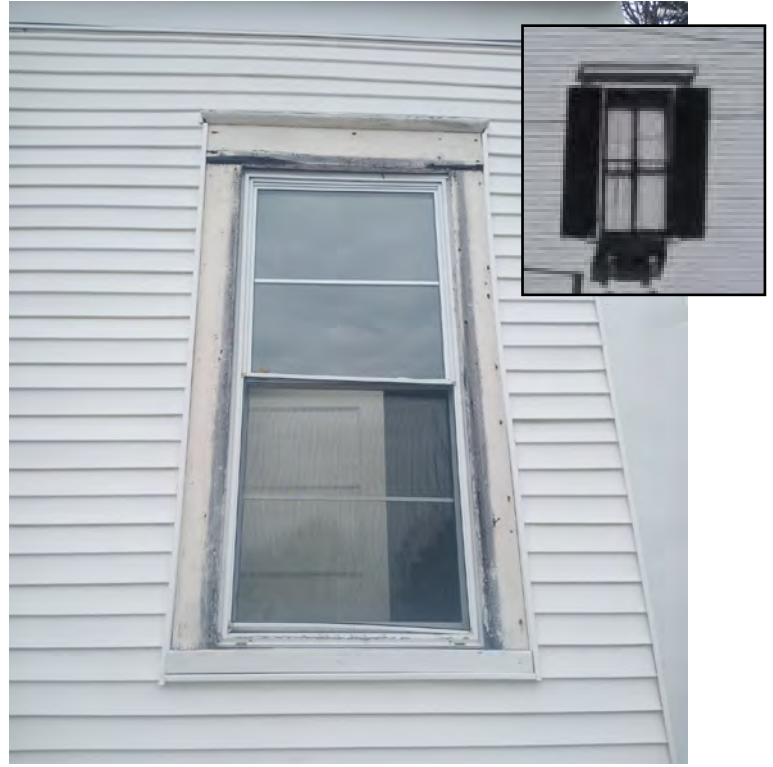
Figure 42: Side façade 1830 window trim; Inset: Windows prior to 1990's were 2/2 double-hung sash (front window pictured). These are thought to have been installed by the Masons in the 1920's.
