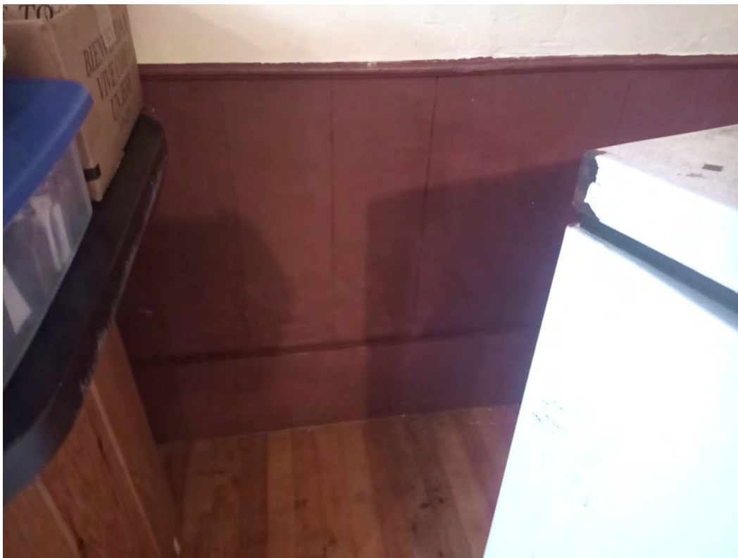
Figure 60: Main hall rear wainscot, wide plank boards
