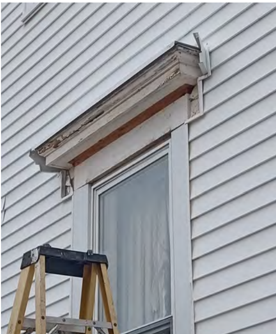
Figure 4: Masonic Hall front window with vinyl siding removed to reveal intact wood window head trim
