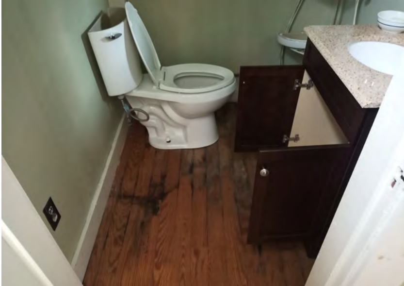
Figure 117: Northeast bathroom – Staining and floor damage
