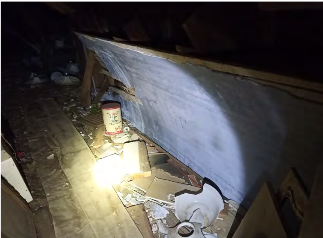
Figure 71: View inside roof eave / attic, note remnant of former blue-painted cove ceiling
