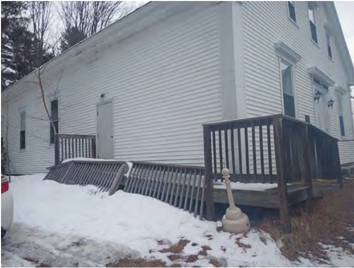
Figure 131: Accessible ramp at west façade requires repair or replacement
