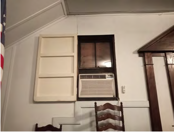
Figures 146-147: Blocked up rear second floor window (2/2 double-hung) with air conditioner unit. AC supports are not safe and should be repaired as soon as possible.
