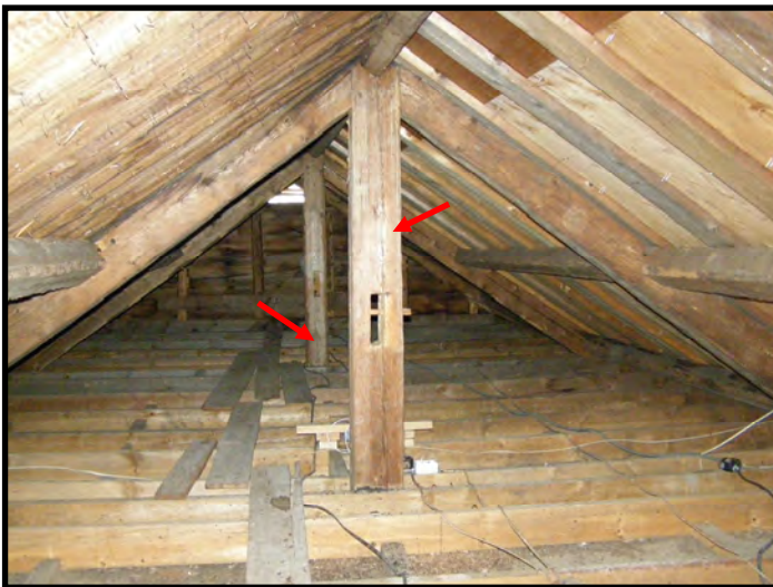
Attic space above second floor at the Masonic Temple. The king posts are indicated in red, these have been cut off the ceiling level, sandwiched and fastened between the 2x6 ceiling joists.
