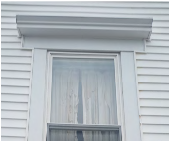
Figure 97: Window head trim with vinyl covering
