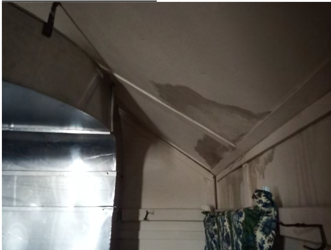
Figure 124: Staining due to water infiltration at second floor ceiling
