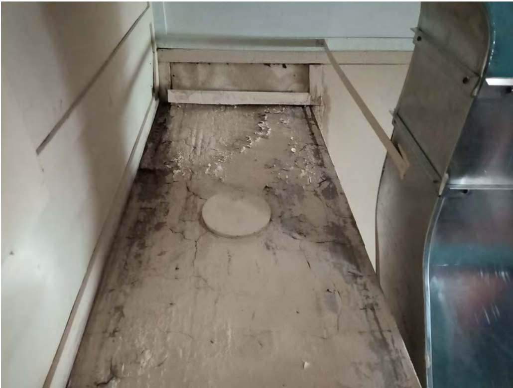
Figure 122: Severe cracked, peeling, bubbling paint due to water infiltration at southeast chimney
