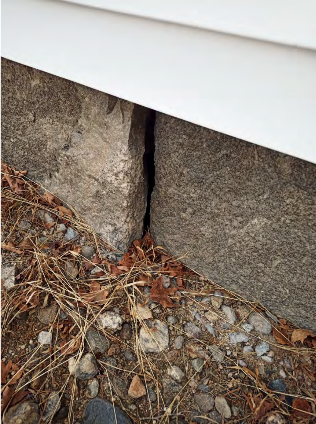
Figure 82: Displacement at split-granite stones, typical
