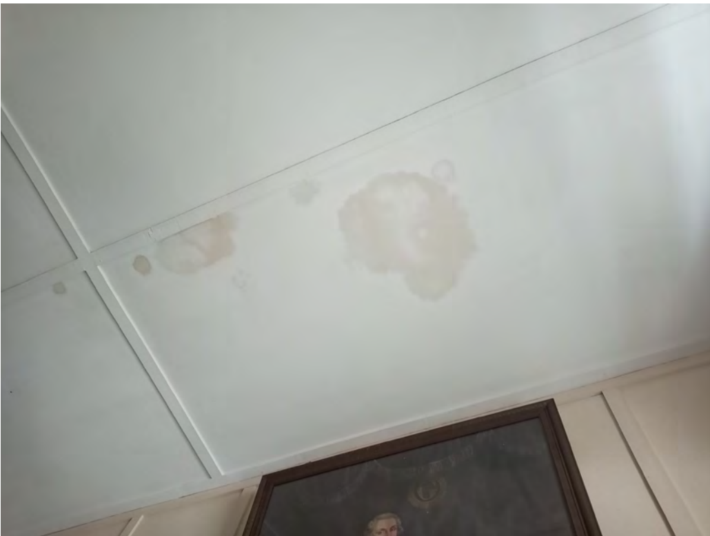
Figure 123: Staining due to water infiltration at second floor ceiling
