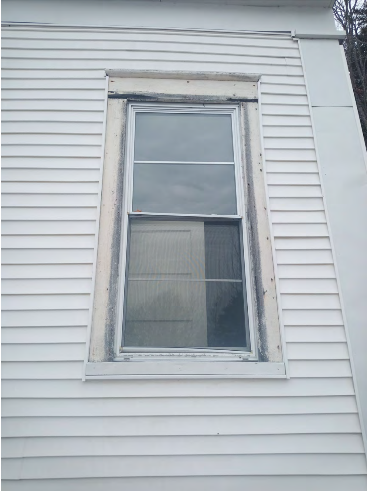
Figure 99: East side window with flat wood trim exposed
