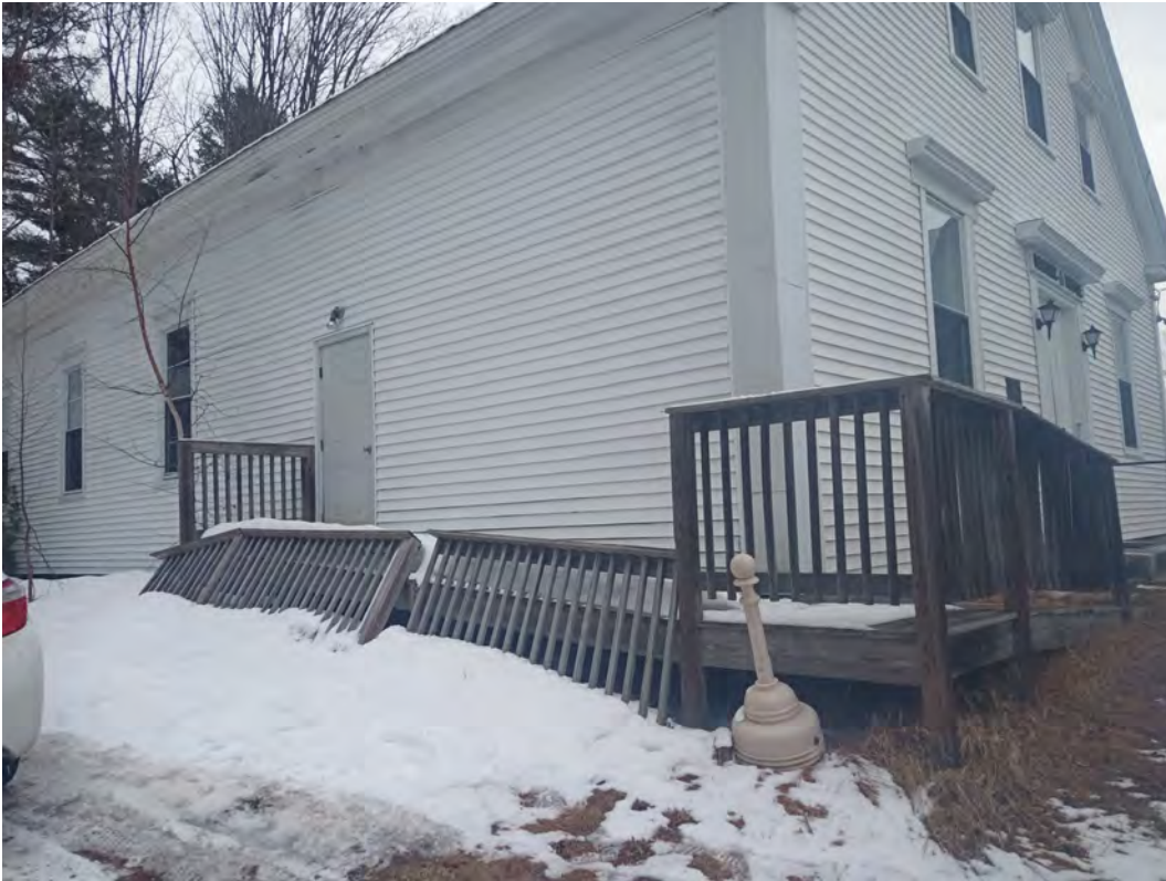
Figure 78: Ramp railing blown off due to snow sliding off roof
