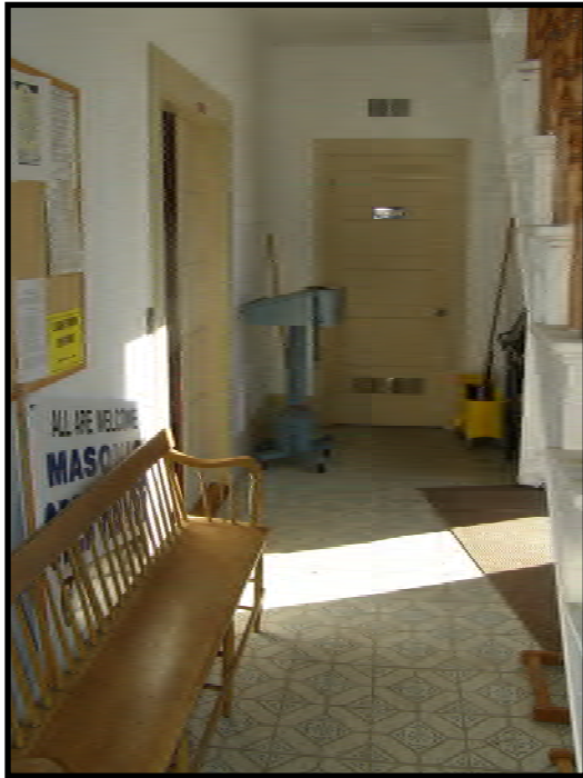
Masonic Temple first floor lobby, looking towards the east. The tile floor in this space has tested positive for asbestos.
