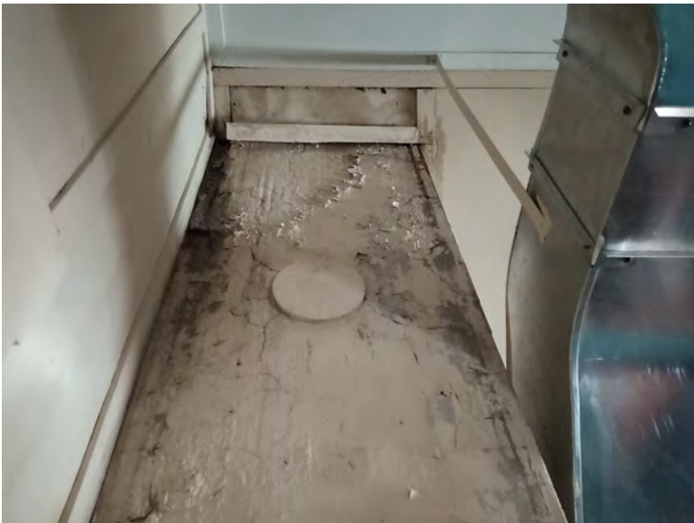
Figure 95: Interior view of chimney & former stove pipe connection
