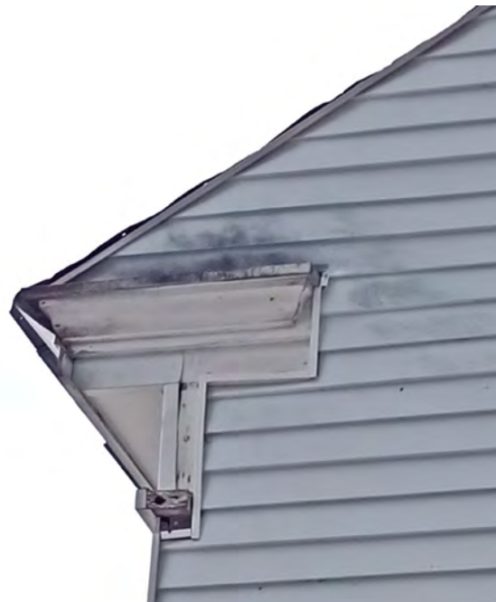
Figure 5: Intact wood cornice / eave trim at northeast corner of building
