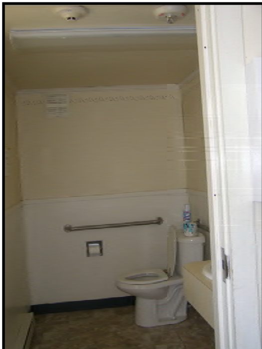
Town Office Restroom. 18" ver. cal grab bar on the sidewall of the toilet required for accessibility is not installed.
