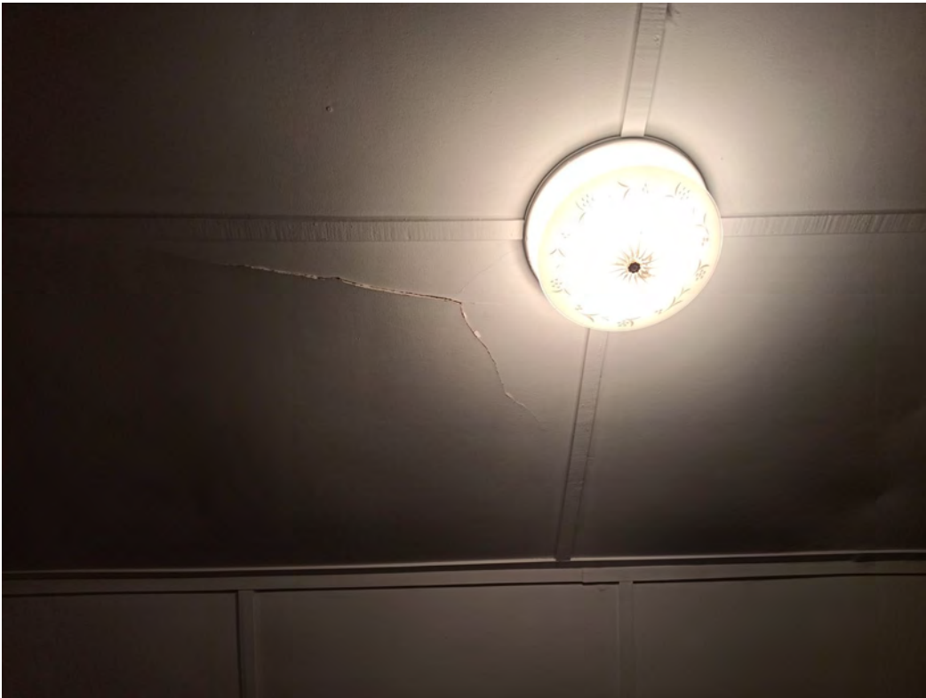
Figure 121: Cracked second floor ceiling finishes
