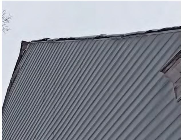
Figure 90: North roof rake, no drip or coverage
