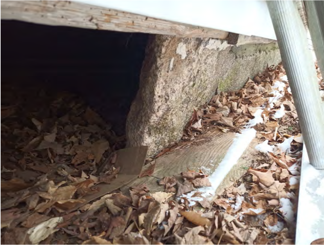
Figure 83: Displacement and cracking at split-granite stones, typical
