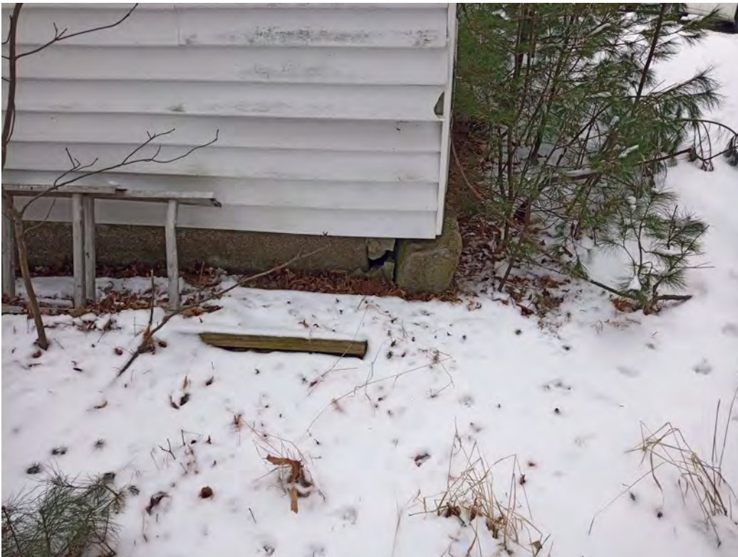
Figure 81: Displacement and cracking at split-granite stones, typical
