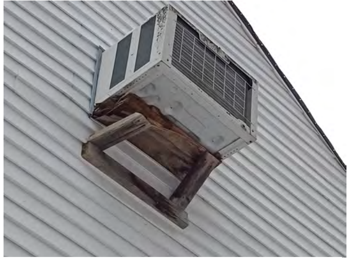
Figures 146-147: Blocked up rear second floor window (2/2 double-hung) with air conditioner unit. AC supports are not safe and should be repaired as soon as possible.
