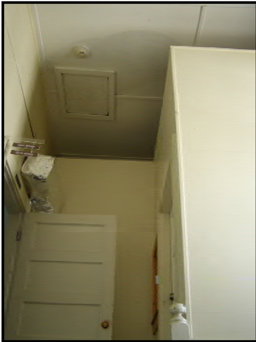
Attic access hatch in ceiling above the second floor stair landing
