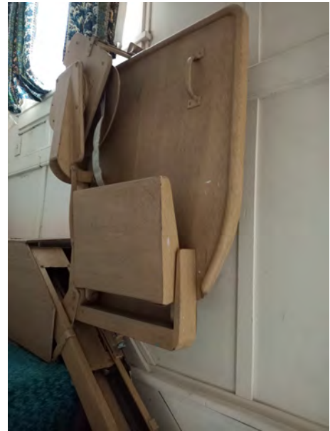
Figures 133 & 134: Access to the second floor is via a wooden stair chairlift that is no longer functional. If replaced in-kind, standby power must be maintained for this to be considered a code-compliant accessible means of egress.
