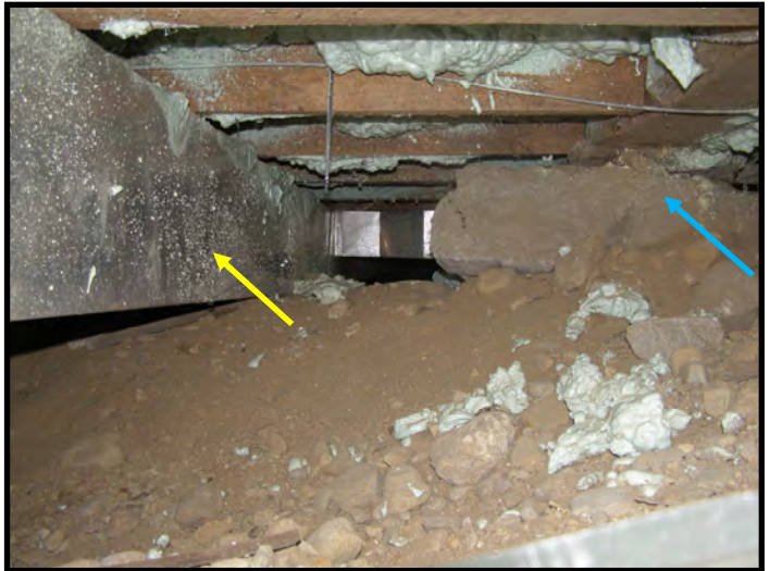
Photo of the first floor system taken from the crawl space. Blue arrow indicates a stone support. The yellow arrow indicates metal distribution ducting for the oil furnace.
