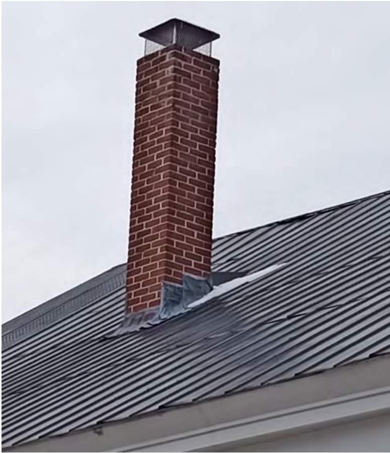
Figure 94: Chimney and step flashing
