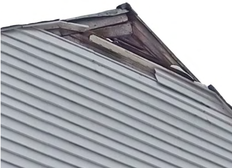
Figure 107: Missing vinyl siding, large opening at rear (north) attic ridge
