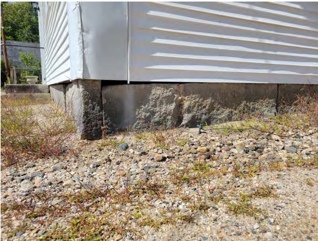
Figure 88: Displacement and cracking at split-granite stones, typical
