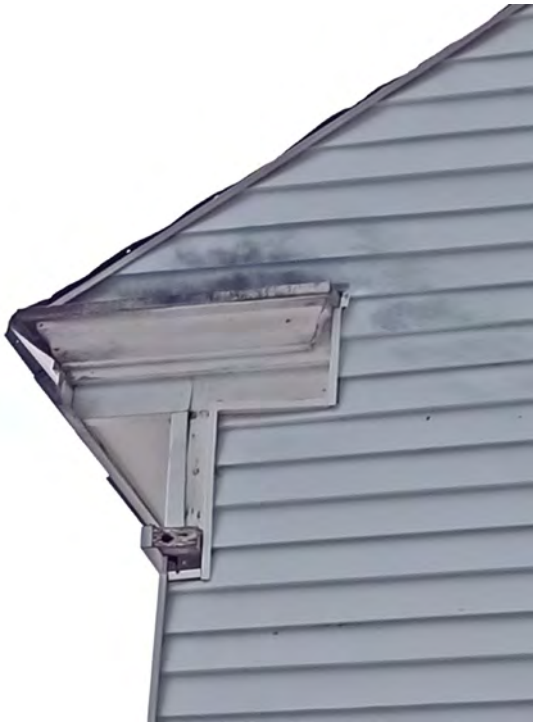
Figure 101: Intact wood cornice / eave trim
