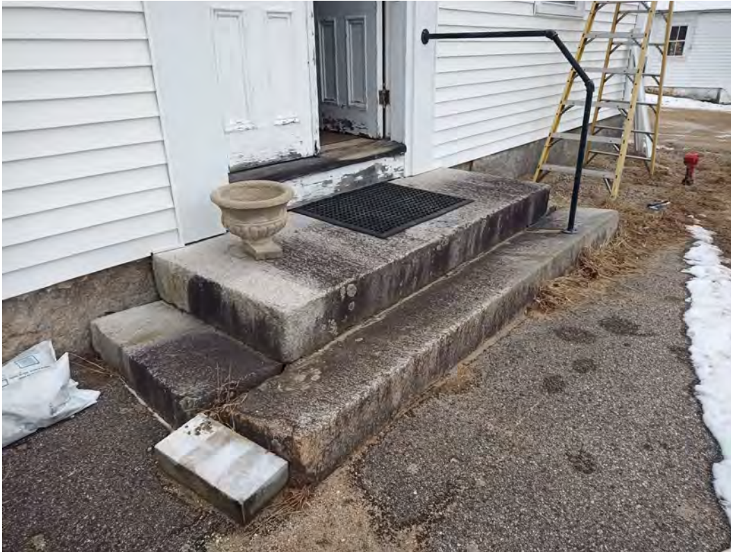
Figure 76: Stone entry steps have sunk with pitch toward building; Stones exhibit staining and biological growth due to moisture accumulation
