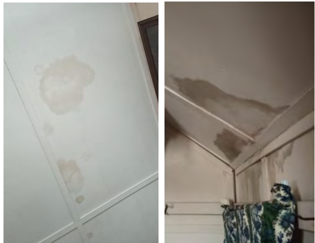
Figures 92 & 93: Staining due to water leaks at second floor ceiling
