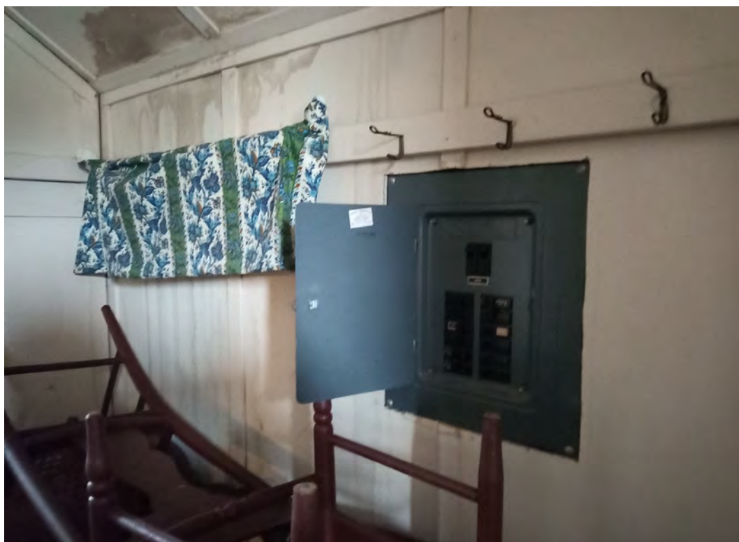
Figure 125: Staining due to water infiltration at second floor ceiling and wall
