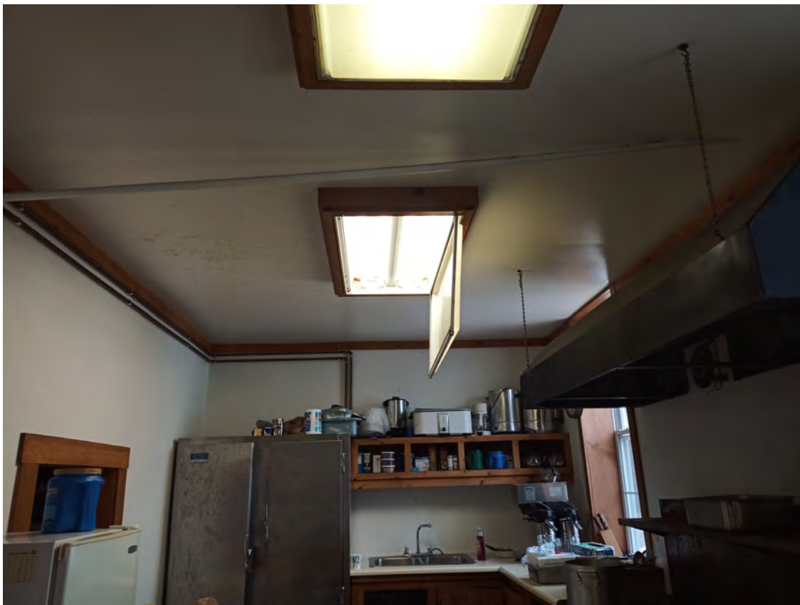
Figure 119: Fluorescent lighting and loose light cover (unsafe) in kitchen
