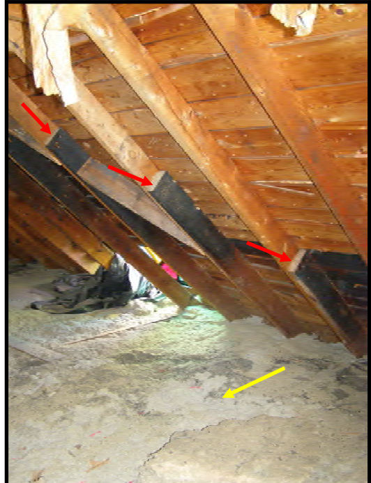
Photo of the attic. Red arrow indicates charred/cut rafters. Yellow arrow indicates blown-in cellulose insulation in the ceiling joist bays
