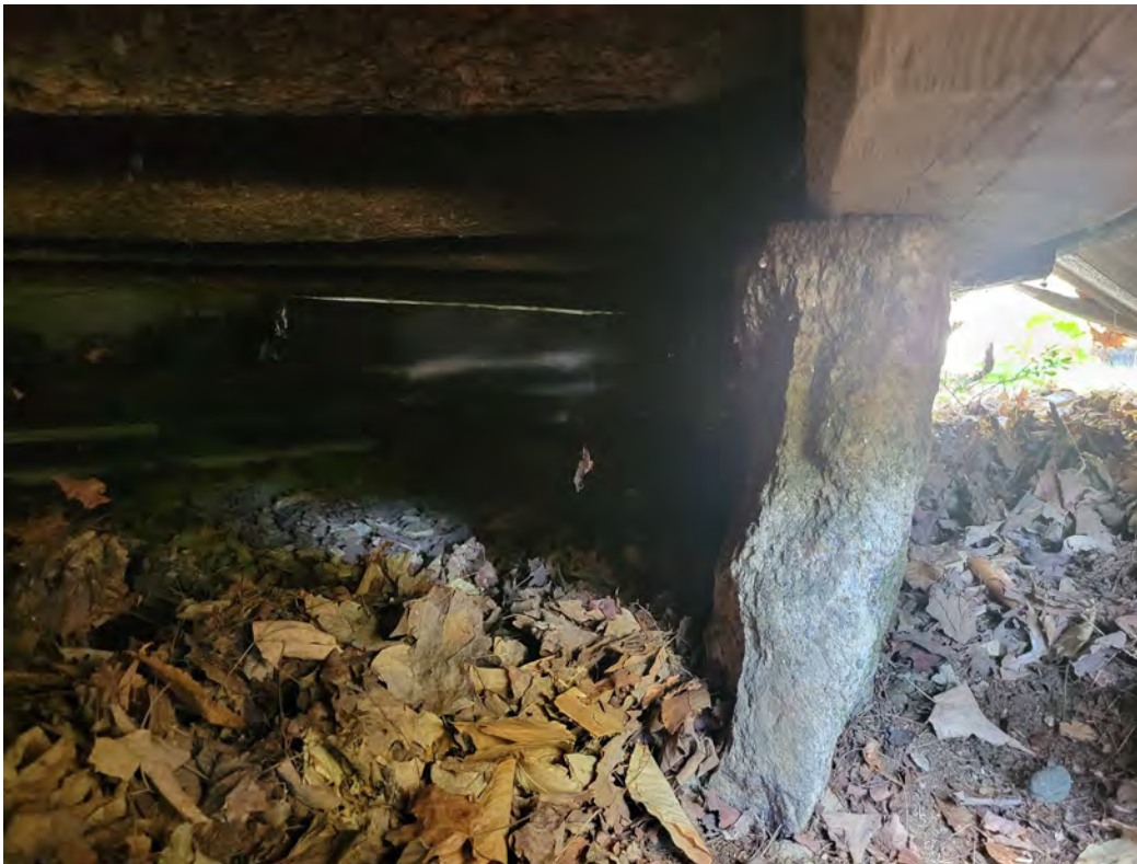
Figure 86: Split granite stone – Reset for full bearing
