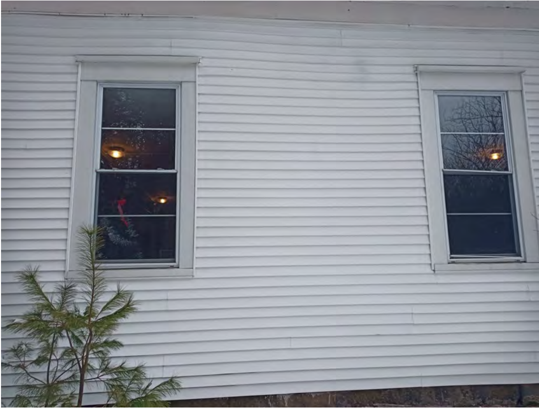
Figure 104: West façade window trim, wood window trim exposed and intact
