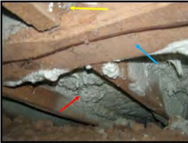
Photo of the first floor system taken from the crawl space. Blue arrow indicates a main carrying beam. The Yellow arrow indicates where the floor joists are 1/2 mortised into the beam. The red arrow indicates where approximately 6" of spray foam insulation has been installed between the floor joist bays.
