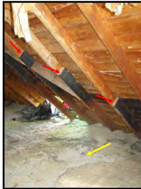
Photo of the attic. Red arrow indicates charred/cut rafters. Yellow arrow indicates blown-in cellulose insulation in the ceiling joist bays
