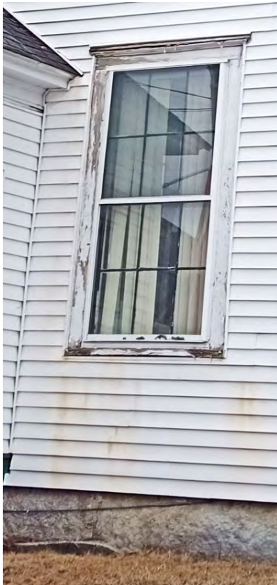
Figure 72: Paint loss, deterioration of wood trim at first floor windows; Staining of vinyl siding
