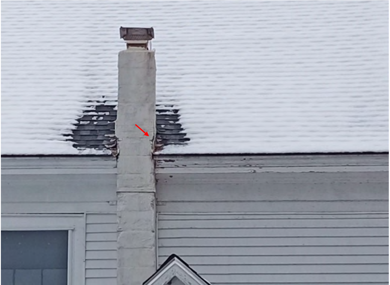
Figure 77: Separation at parging; Paint loss and deterioration at wood eave trim; Openings at step flashing.
