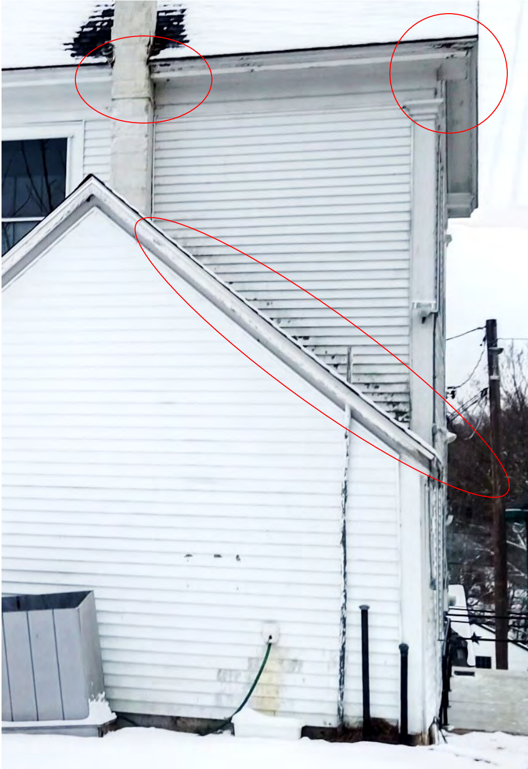
Figure 74: Paint loss and deterioration of wood trim at eaves and rake; Staining at vinyl siding.
