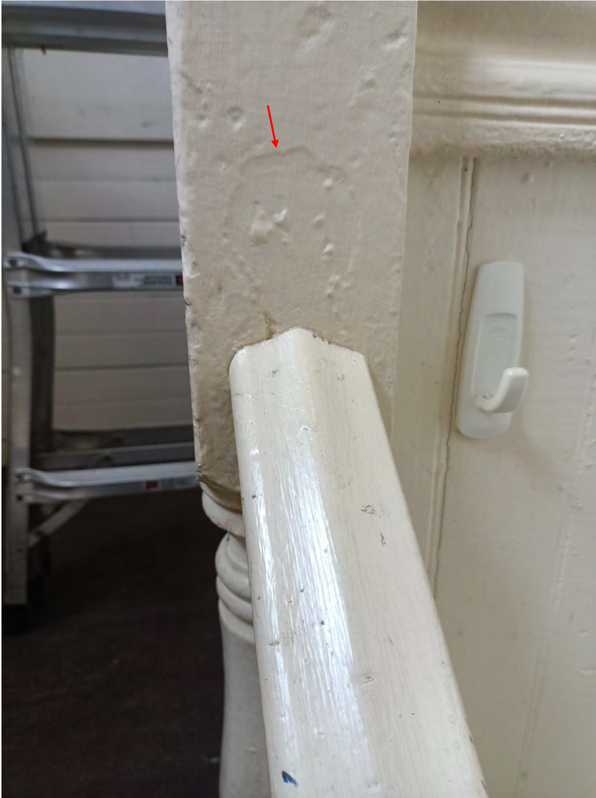
Figure 53: Detail view of stair handrail; Note possible ghost / outline of previous rail.
