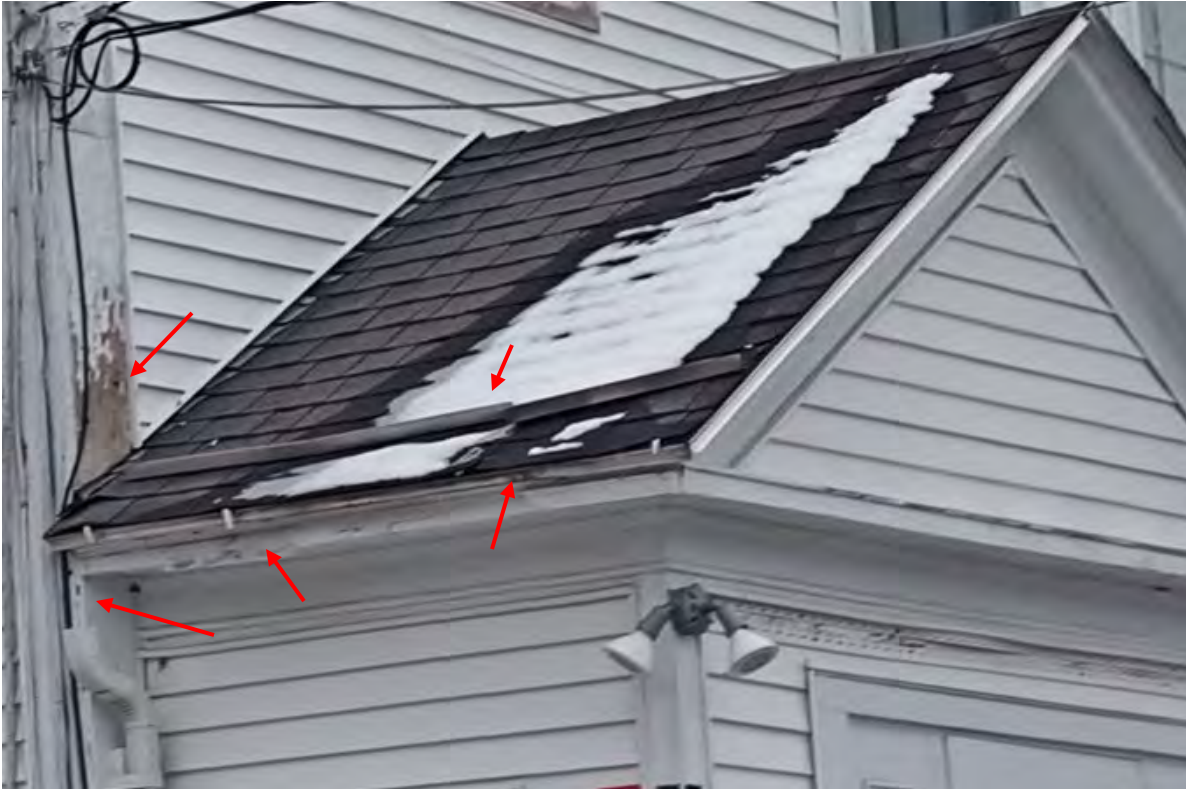
Figure 80: Non-functioning diverter causing deteriorated trim; Downspout elbow with no gutter.
