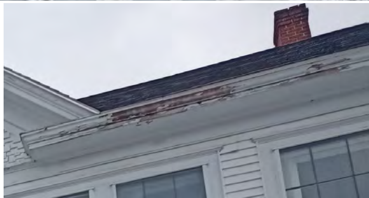
Figures 69 & 70: Paint loss, rotted wood trim at eaves beneath valleys
