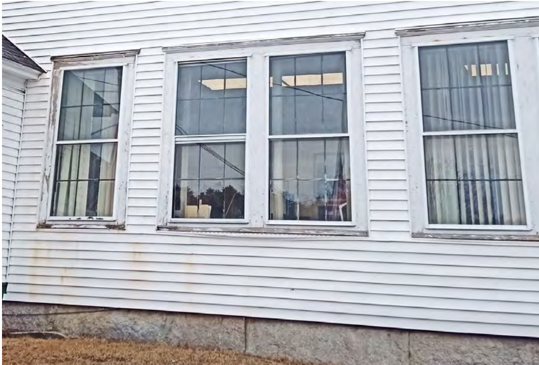
Figure 71: Paint loss, deterioration of wood trim at first floor windows
