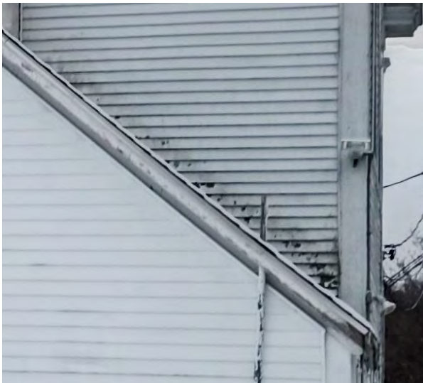
Figure 78: Staining and biological growth along addition roof indicates inadequate flashing, standing snow, poor drainage, and/or saturated shingles causing moisture to wick up wall. Rotted wood likely to be found behind siding.
