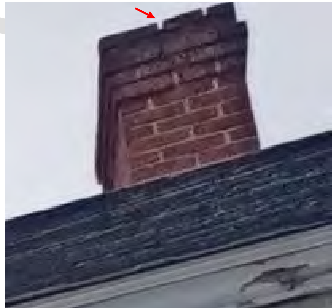
Figure 79: Open mortar joints at corbelled chimney top; Deteriorated wood trim in foreground.
