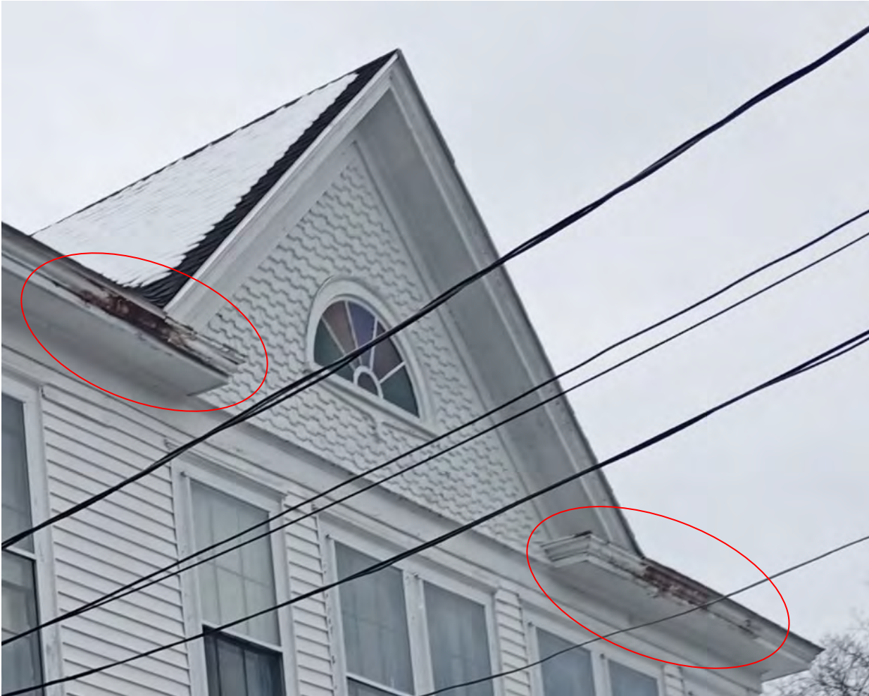
Figures 69 & 70: Paint loss, rotted wood trim at eaves beneath valleys
