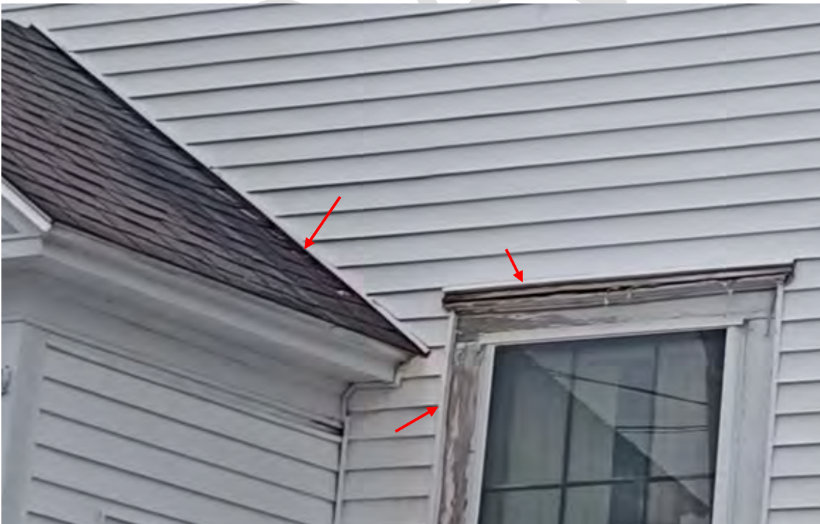
Figure 81: Roof run-off causing localized severe deterioration of window trim. Diverter or gutter sloped to exterior would be useful here and there should be a minimum 4" gap from shingles to bottom of siding with metal step flashing.
