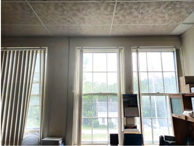
Figure 88: First floor office features outdated textured acoustic tile suspended ceiling and vertical blinds, which are not ideal for south windows.
