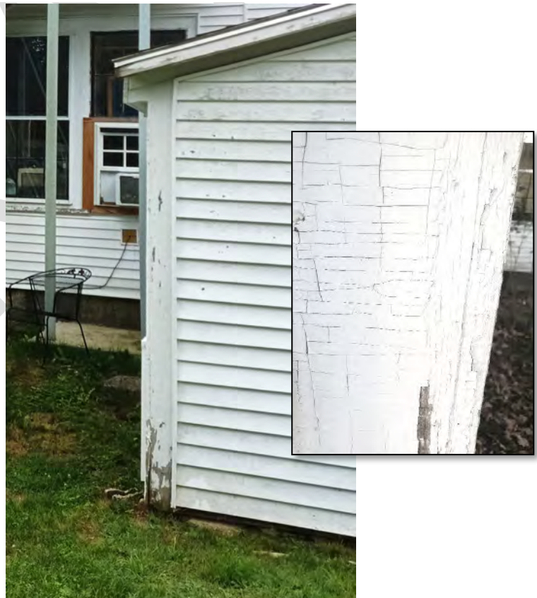
Figure 73: Paint loss, deterioration of wood corner trim rear addition; Inset: Example of crazed lead paint at corner trim
