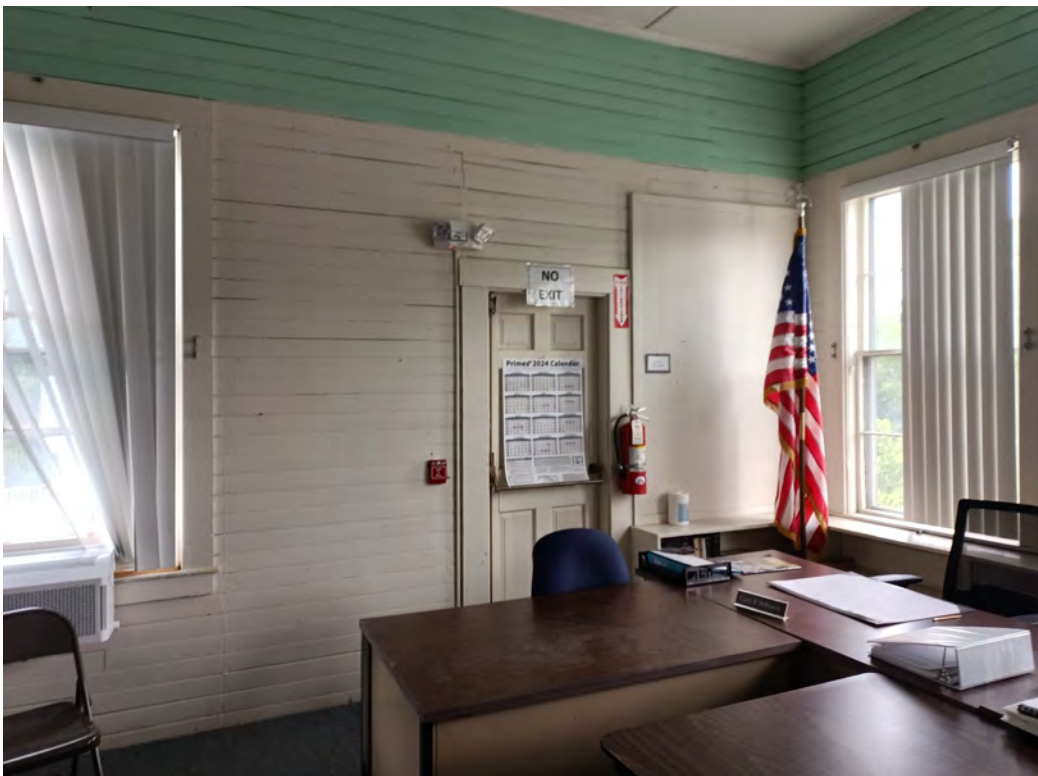
Figure 65: View of five-panel door that previously led to east second floor fire escape
