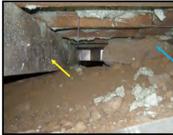
Photo of the first floor system taken from the crawl space. Blue arrow indicates a stone support. The yellow arrow indicates metal distribution ducting for the oil furnace.
