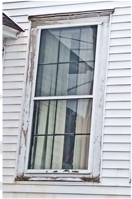
Figure 83: Typical original (1895) 6/6 double-hung window
